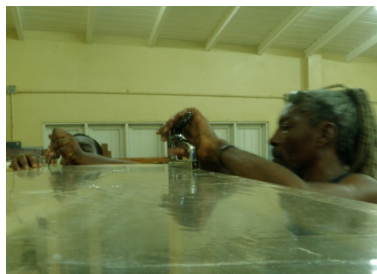
7. Pull plastic tight around and staple onto frame
